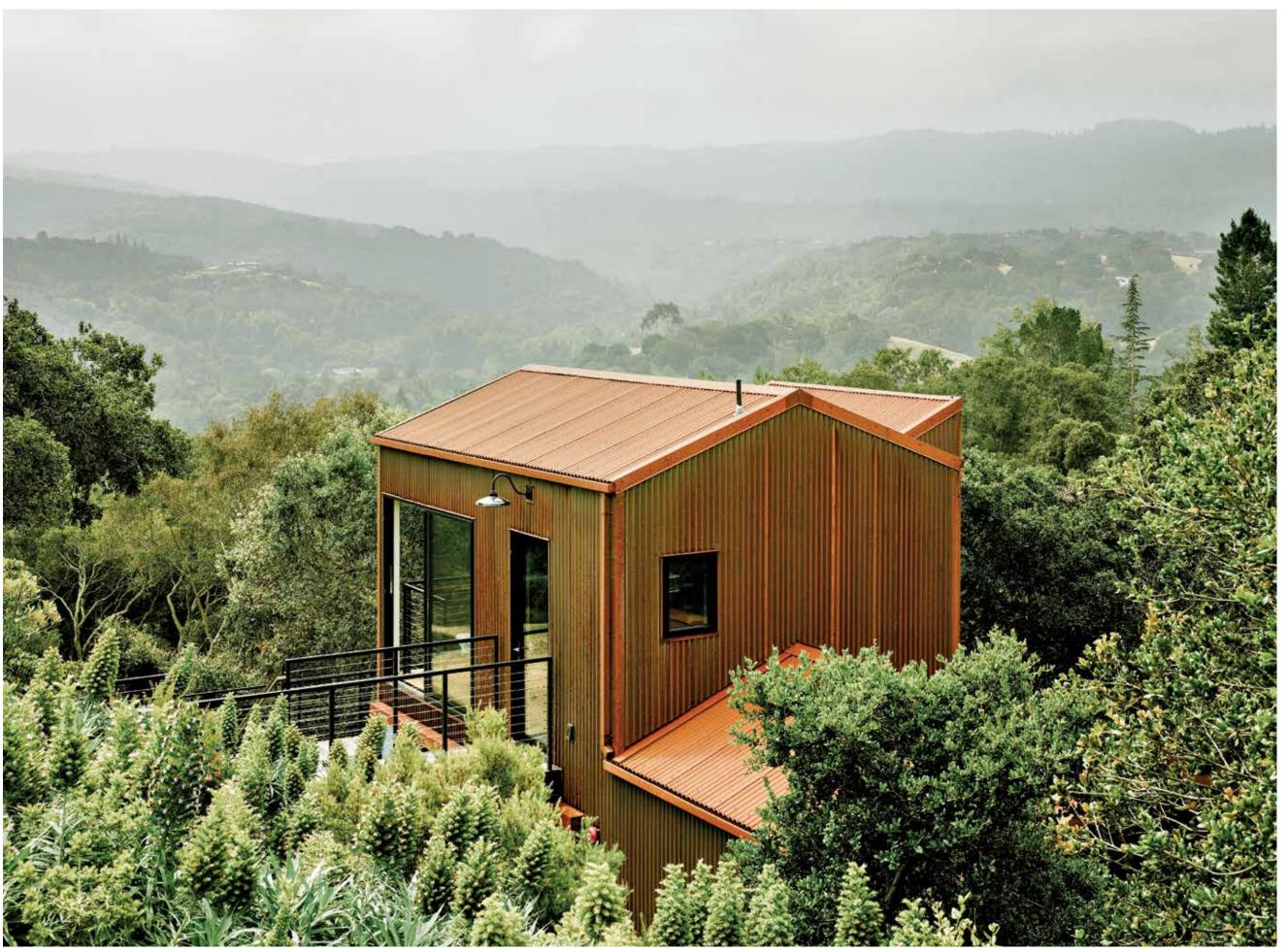
The roof and exterior of the guesthouse are clad with Cor-Ten corrugated steel, installed by Bill Hamilton Roofing, to evoke the area's agricultural buildings. A bridge connecting the building to the main house was fabricated by Bob's Iron. The property's new landscaping was designed by Randy McDannell and installed by Elements Landscape.
